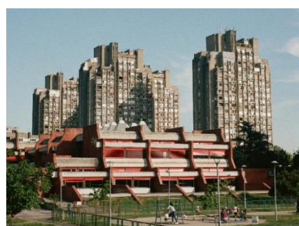
Figure 13: Block 23 high rise housing buildings (26)
