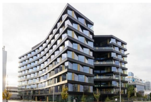
Figure 17: Non-residential /office building GTC X (2022) (30)
